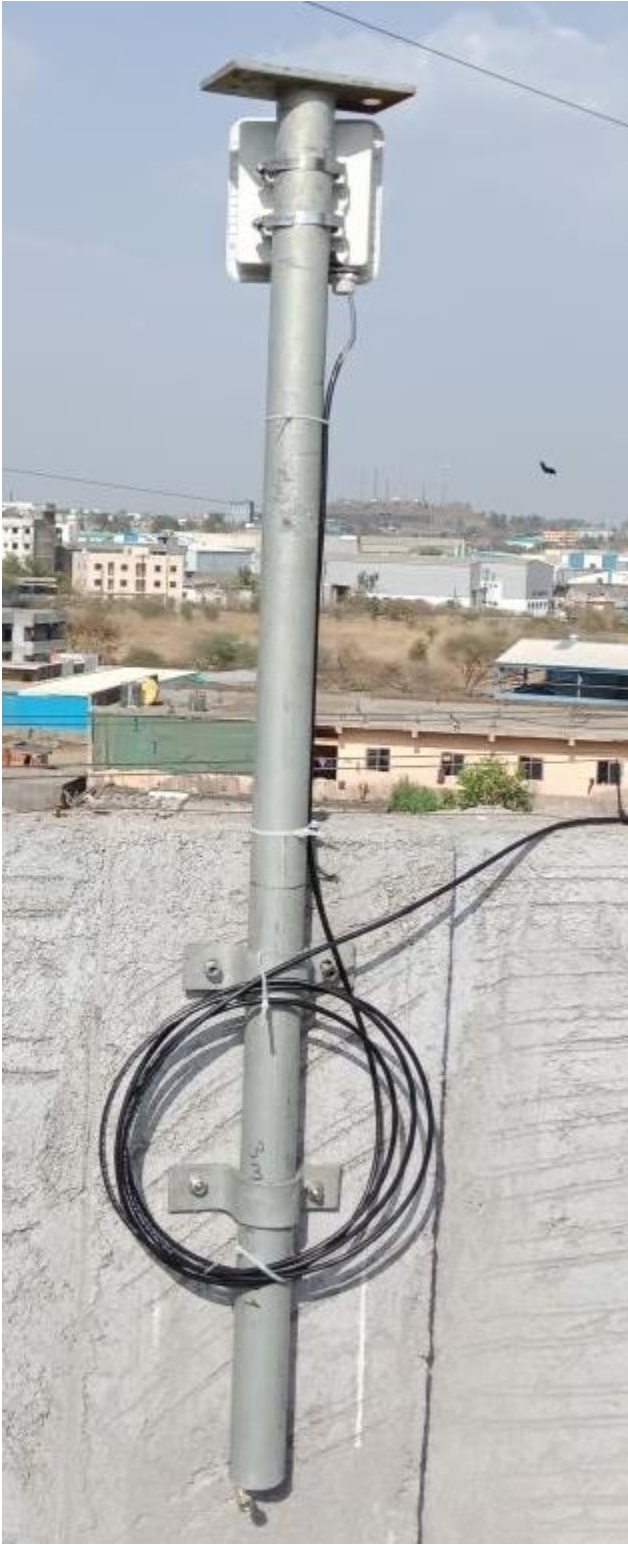
Pole Mount Router Installation picture:
